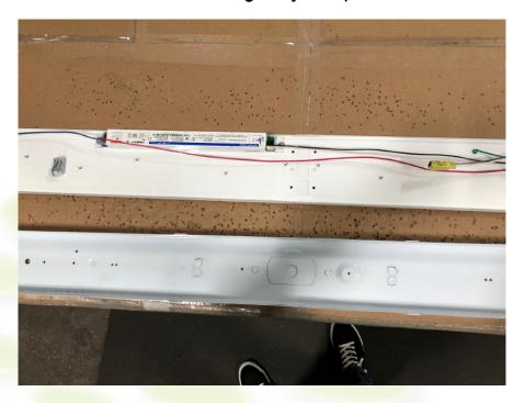
2. Quick Connect the LSR retrofit to the old strip's disconnect, and place the LSR over the strip housing.
