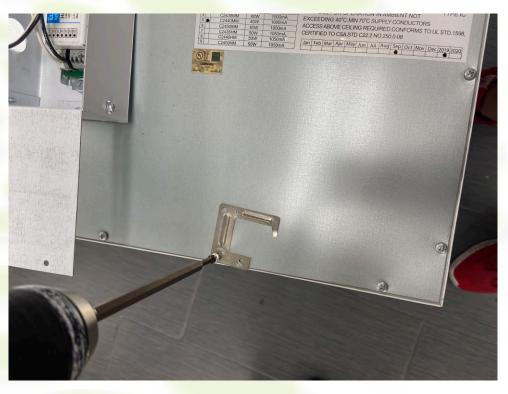
Step 6: Place the new pre-wired driver box underneath the earthquake clips, and then re-attach the earthquake clips. Installation is complete.
