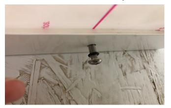
3. Slide lens diagonally into one end of the fixture, then push down and slide to the other end and align holes
